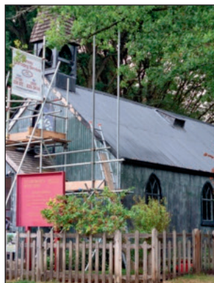
Church repairs. Photo: Angela Stockbridge
